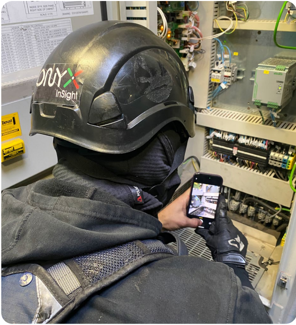
Figure 2: Field engineer completing an inspection using the fieldPRO phone app
