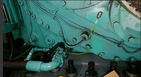
ecoCMS accelerometers retrofitted to GE1.5 MW gearbox
