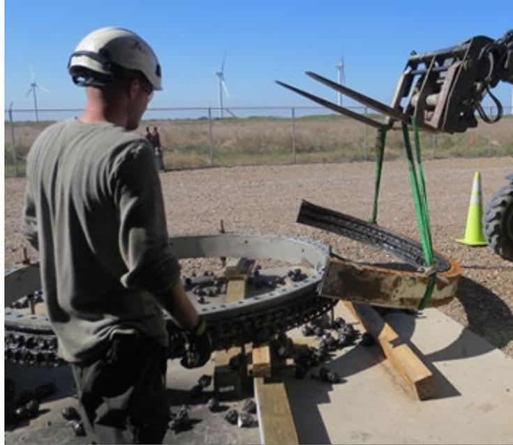
ONYX INSIGHT PROVIDES ROTATING MACHINERY SUPPORT TO PATTERN, SUCH AS PITCH BEARING TEARDOWN PROCEDURES AND GEARBOX PROCUREMENT SPECIFICATIONS
